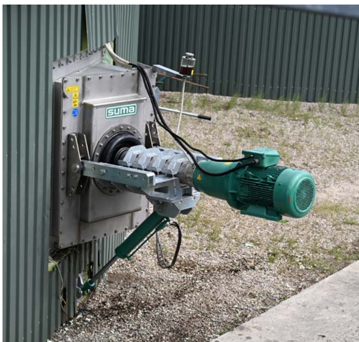
FTX - Concrete tank
