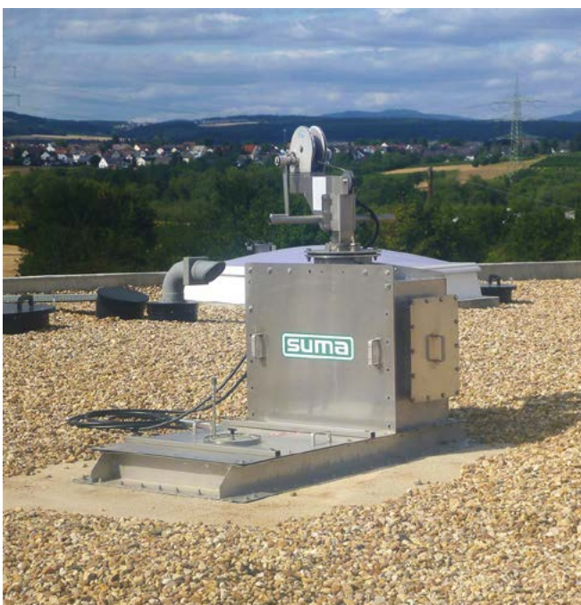
GDD - Concrete tank
