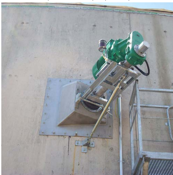
FR 30° - Concrete tank
