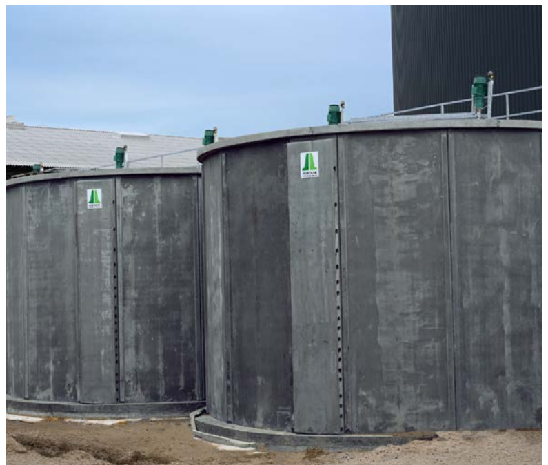
BG2 top mounting - Concrete tank
