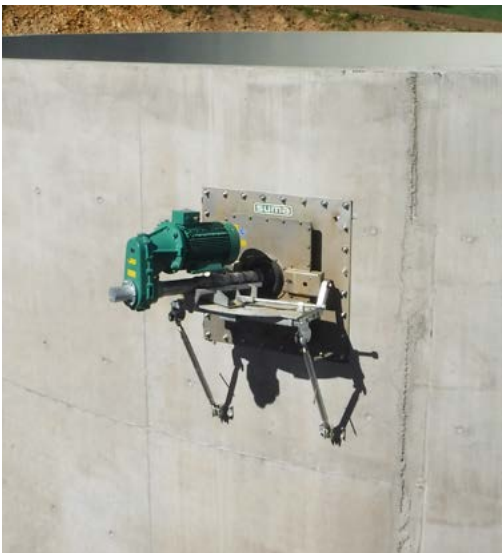
FR SP - Concrete tank
