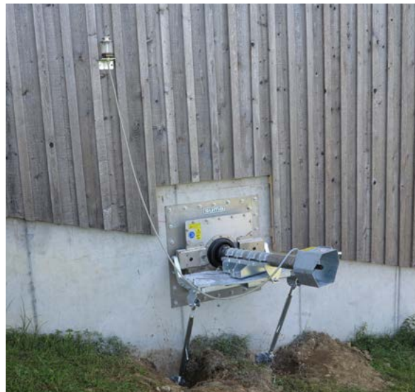
FR SP HY - Concrete tank
