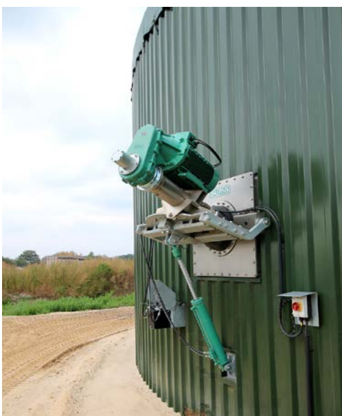
FT - Concrete tank
